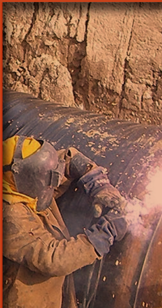
Maintenance, Shutdowns & Turnarounds
